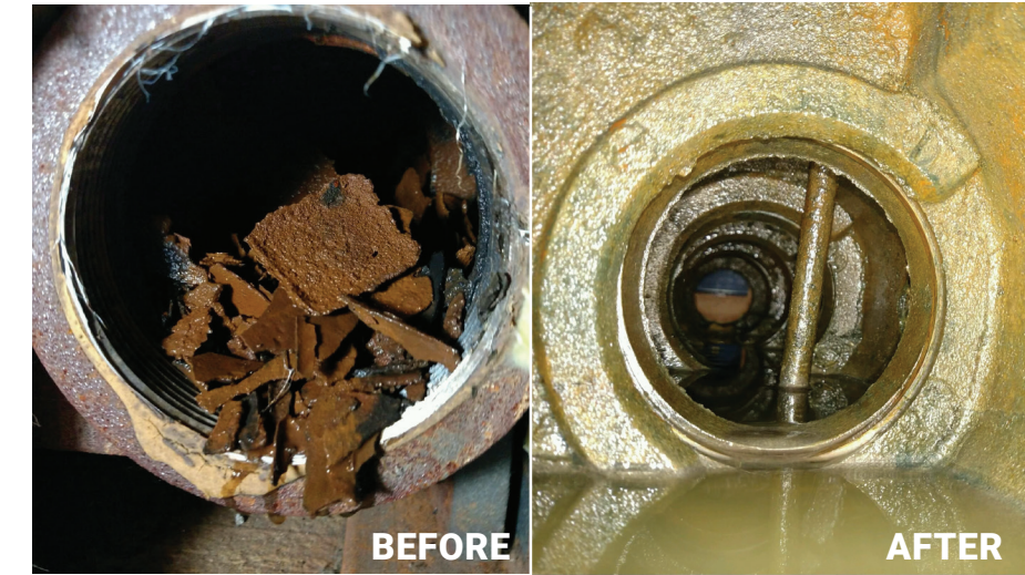
Internal inspection of a cast iron boiler before and after descaling.
